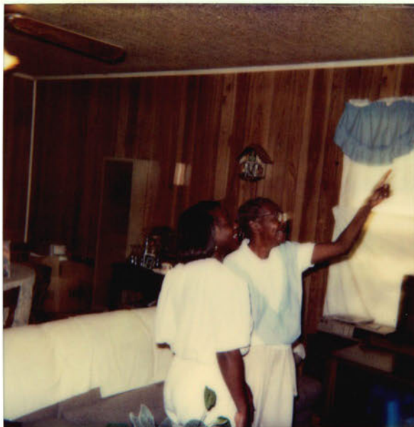
Sheila Lyons helps inspect a home in Ferriday, LA. The customer is hoping to get a loan or grant to repair her home.
