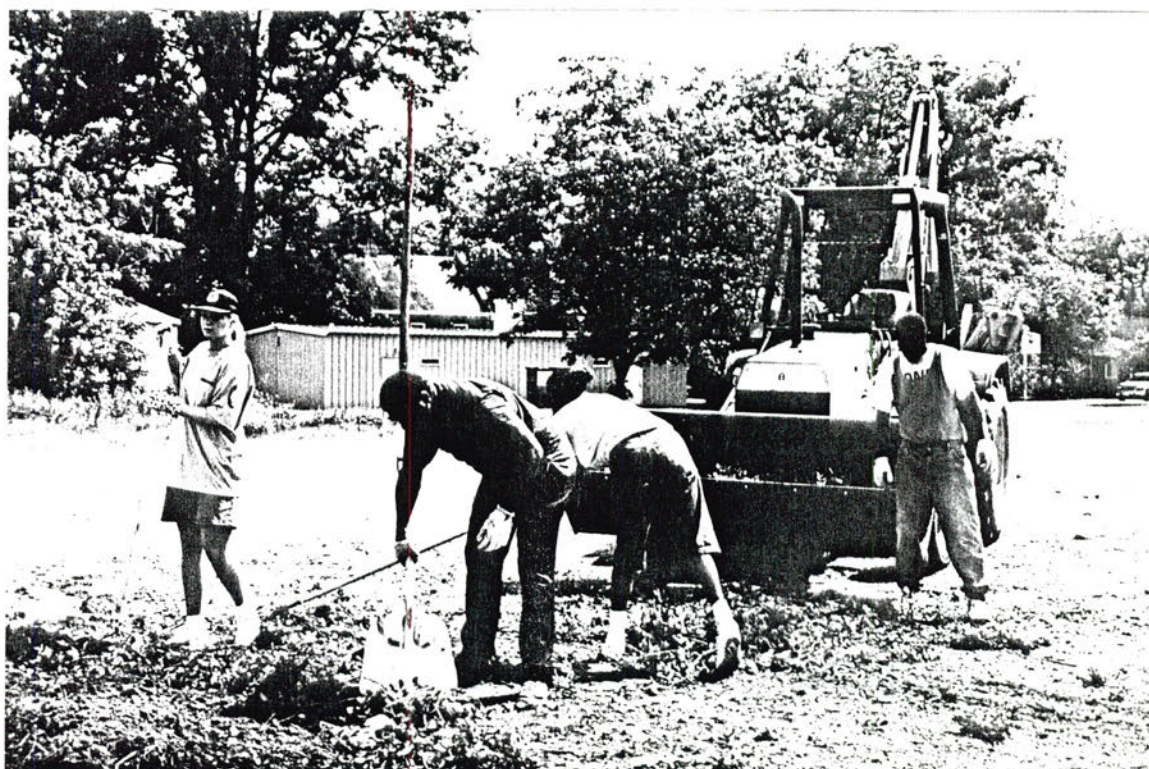
HOLLY GROVE SITE - X05A & Y05A THE "BENT RAIL" DEPOT FUTURE MUSEUM AND GIFT SHOP AmeriCorps members Linda Knox, Leroy Foster, Gloria Wiley, Jana Coleman and James Stewart are working together to enhance the property and building which is on the National Register of Historic places.
