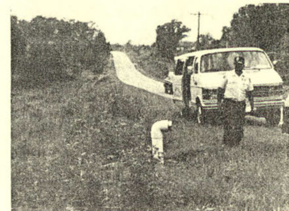
Dry hydrants should be easily accessible.
