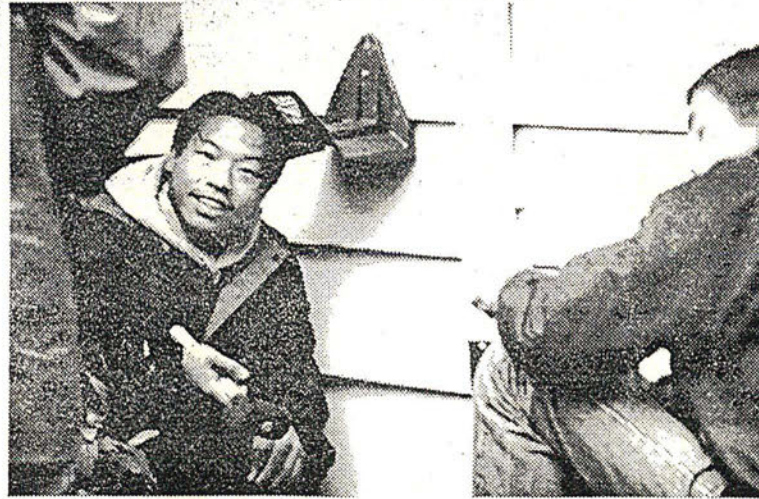
EnviroCorps member Cheng Cha disconnects a downspout in Northeast Portland to help keep pollution out of the Columbia Slough.
