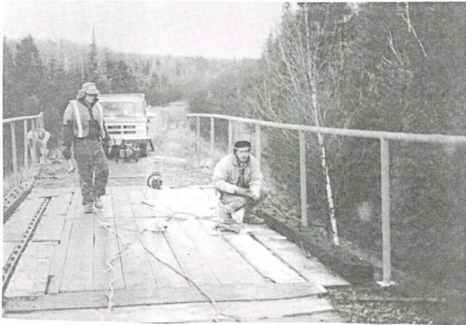
Bridges (above and below) under construction on the Aroostook Valley trail.
