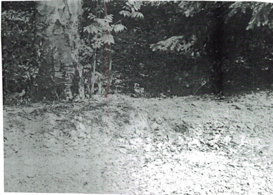
Newly constructed gravel diversion on Barn Brook Road diverts road runoff to vegetated buffer strips.
