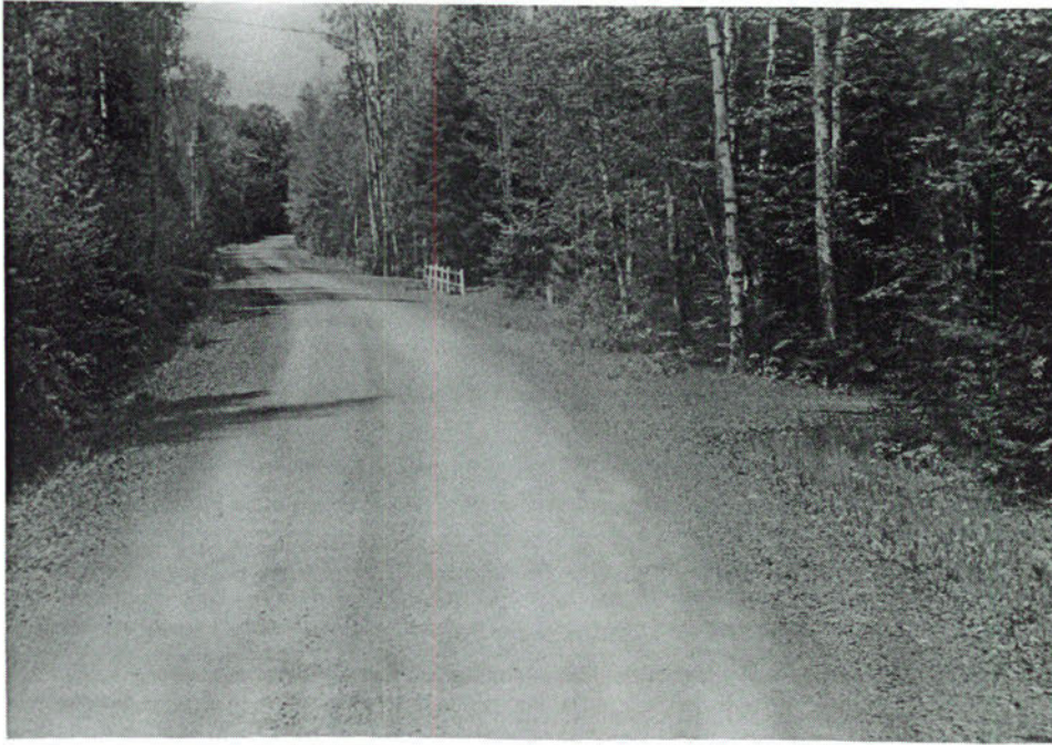
Barn Brook Road on Long Lake after the road is crowned to divert runoff.
