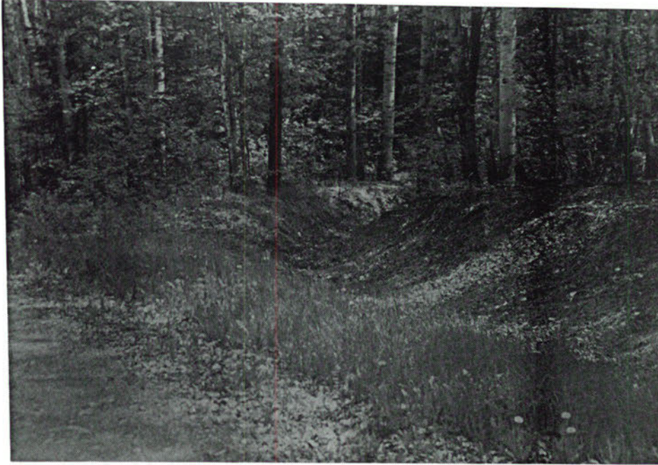
Vegetated buffer strip and newly constructed grassed waterway divert water from a steep hill on Barn Brook Road.
