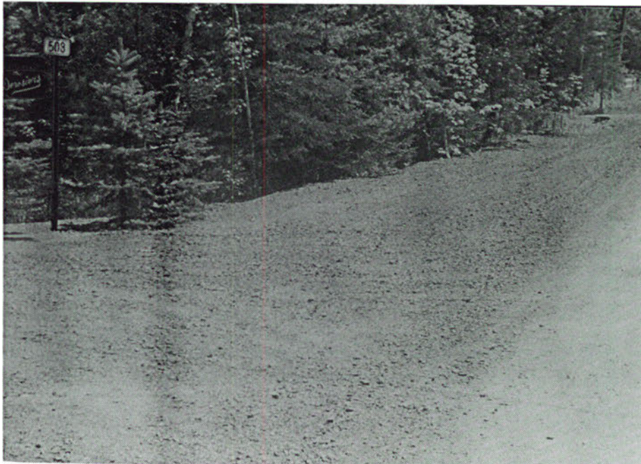
Numerous small road diversions divert runoff to vegetated filter strips.
