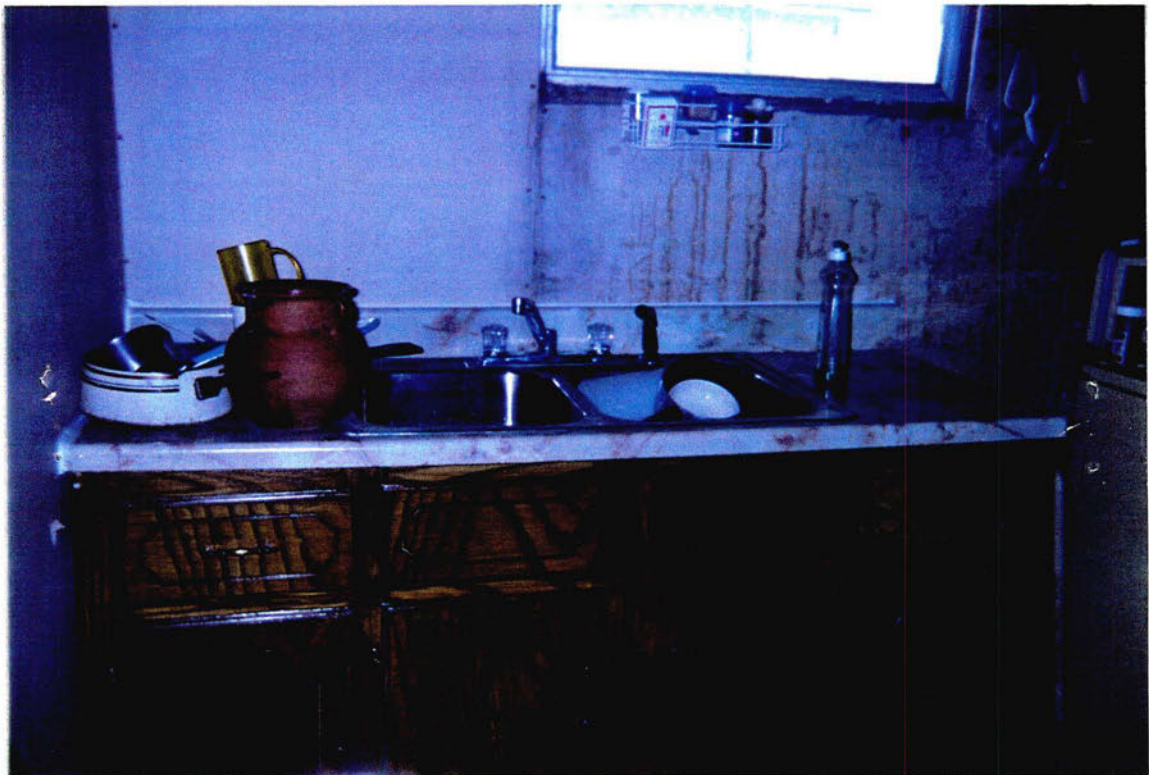
Indoor Plumbing and Running Water Obtained for the Ochoa Family by USDA AmeriCorps Member Serving in South Texas
