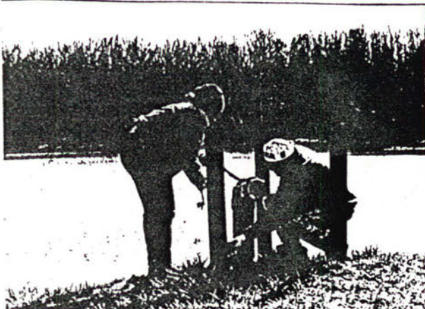
Newberry II members Angela Brinkley(left) and Jay Henderson, both of Columbia, paint a dry hydrant in Richland County.
