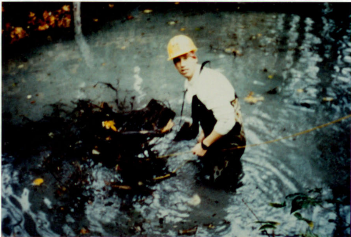
Members place root wads in Gamm Creek overwintering ponds, Quilcene Ranger District, Olympic National Forest. Root wads provide hiding cover for young Chinook and Coho salmon fry.
