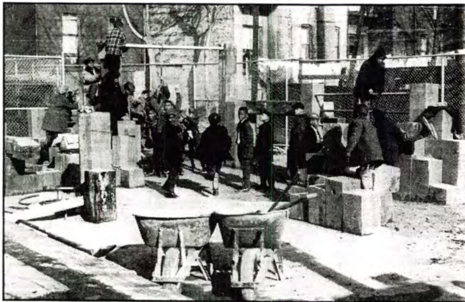
Pratt helps create a park: In addition to building housing, Pratt constructed this early vest-pocket park in Bedford-Stuyvesant.
