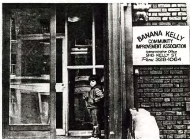
This boy will live in one of the newly renovated apartments on Kelly Street.
