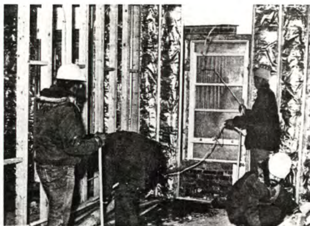
CETA workers installing insulation at Banana Kelly.
