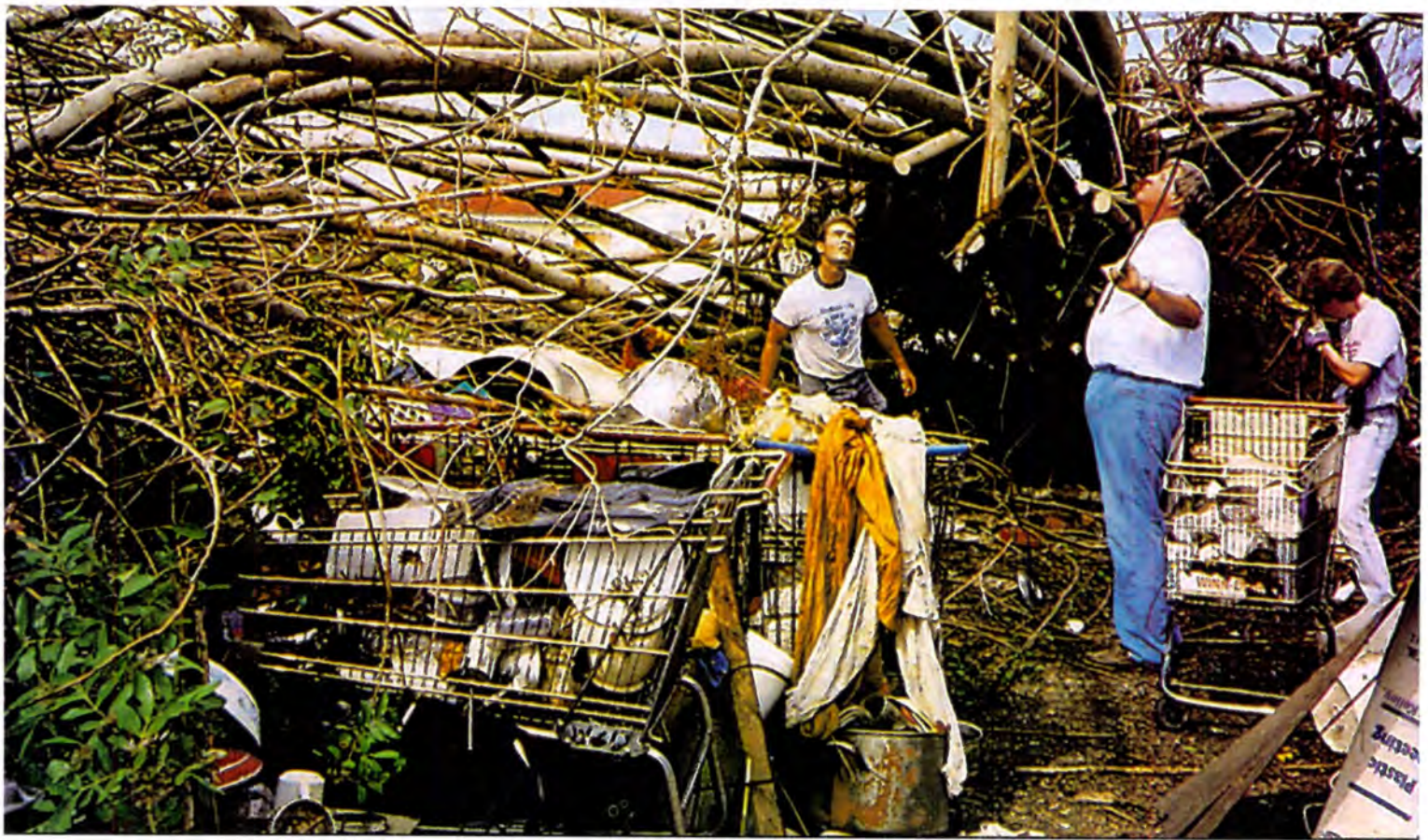
Broward Community College volunteers clear debris for a homeowner in hurricane-ravaged Florida City.
