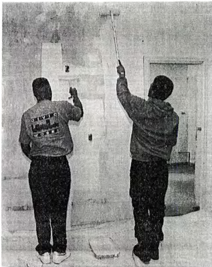
Some of Civic Works' 25 participants repaint the Clifton Mansion.
