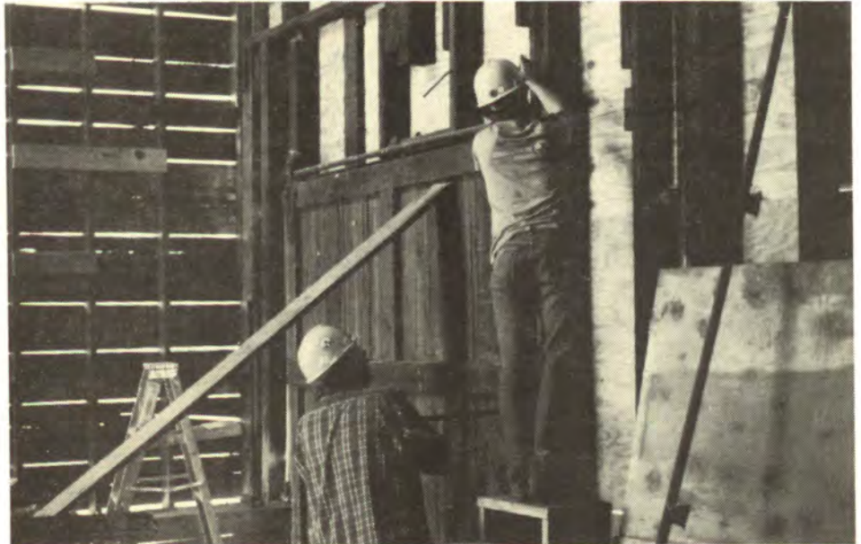
During the restoration process great care was taken not to damage any of the materials that would be reused to maintain historical accuracy.
