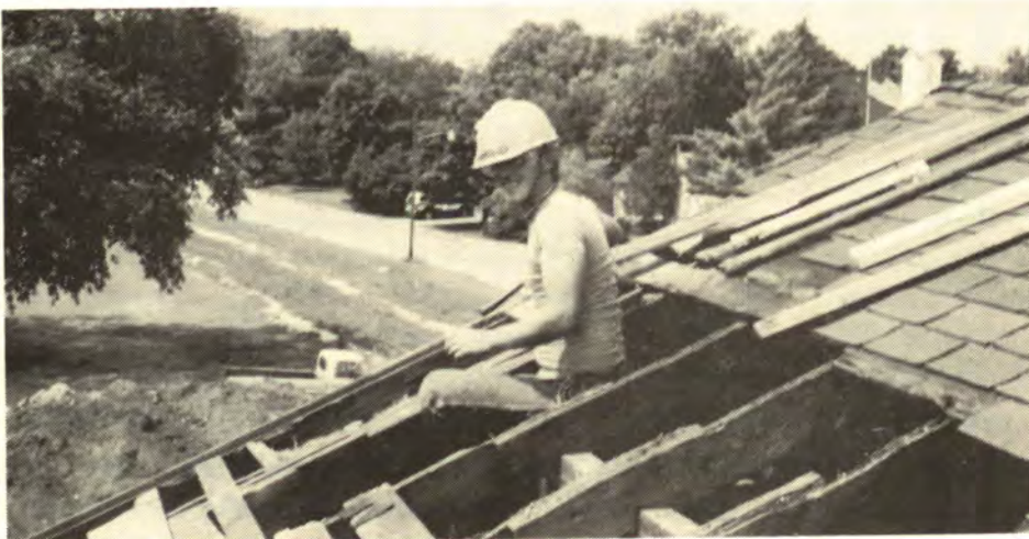
Mazomanie Historical Society Crew Member Jim Horner works to remove sections of the old roof. Members of the Sauk County Crew assisted with the reroofing.
