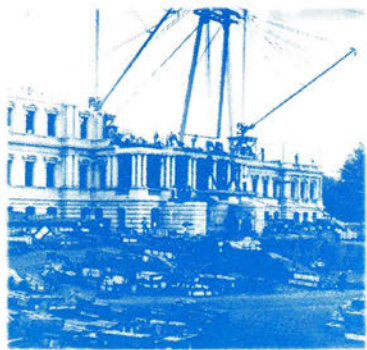
▲ South Wing Construction, June 1873 (Library of Congress)
