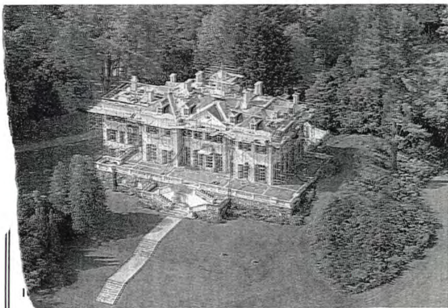
Photograph by Jonas Dovydenas of Lenox, chairman of the board of directors of Edith Wharton Restoration, shows the restoration of The Mount in progress. Wharton lived at The Mount from 1902 to 1911.
