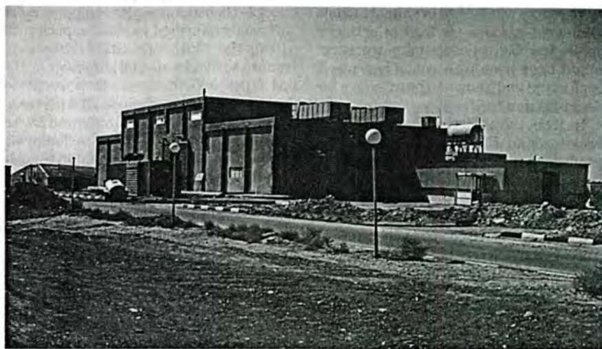
Figure 2.—Main facility for the production of biological warfare agents at Al Hakam Single-Cell Protein Plant (destroyed in June 1996). (Photo courtesy of UNSCOM.)
