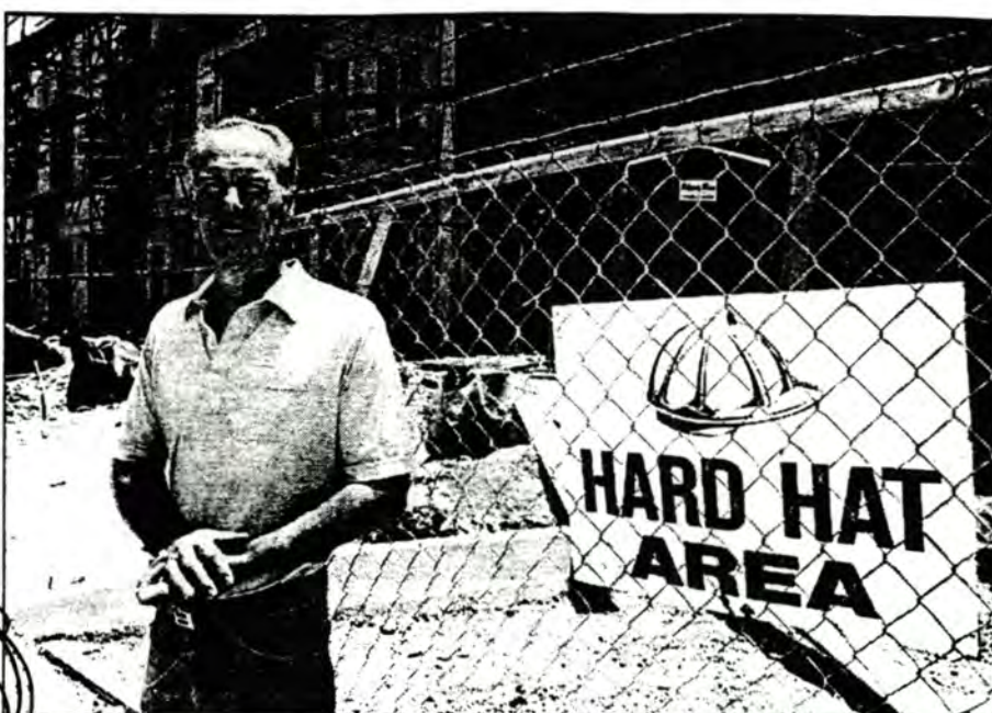
THEY TOOK OVER: Terry Angel, a contractor, says immigrants' cheap labor is forcing Americans out of work. He says illegal aliens work at this Cypress, Calif., building site.
