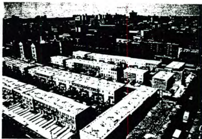
In less than six years the same land was packed with new dwellings, including a number of small family homes.
