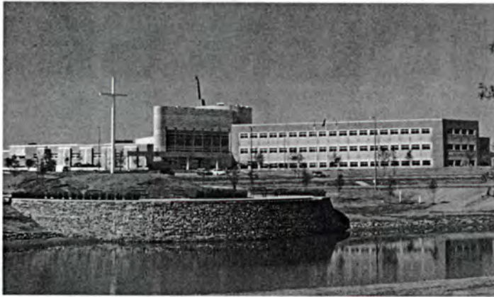
Located on a 157-acre campus, the new Baptist Health Baptist Memorial Medical Center in North Little Rock represents a major addition to Greater Little Rock's healthcare industry.
