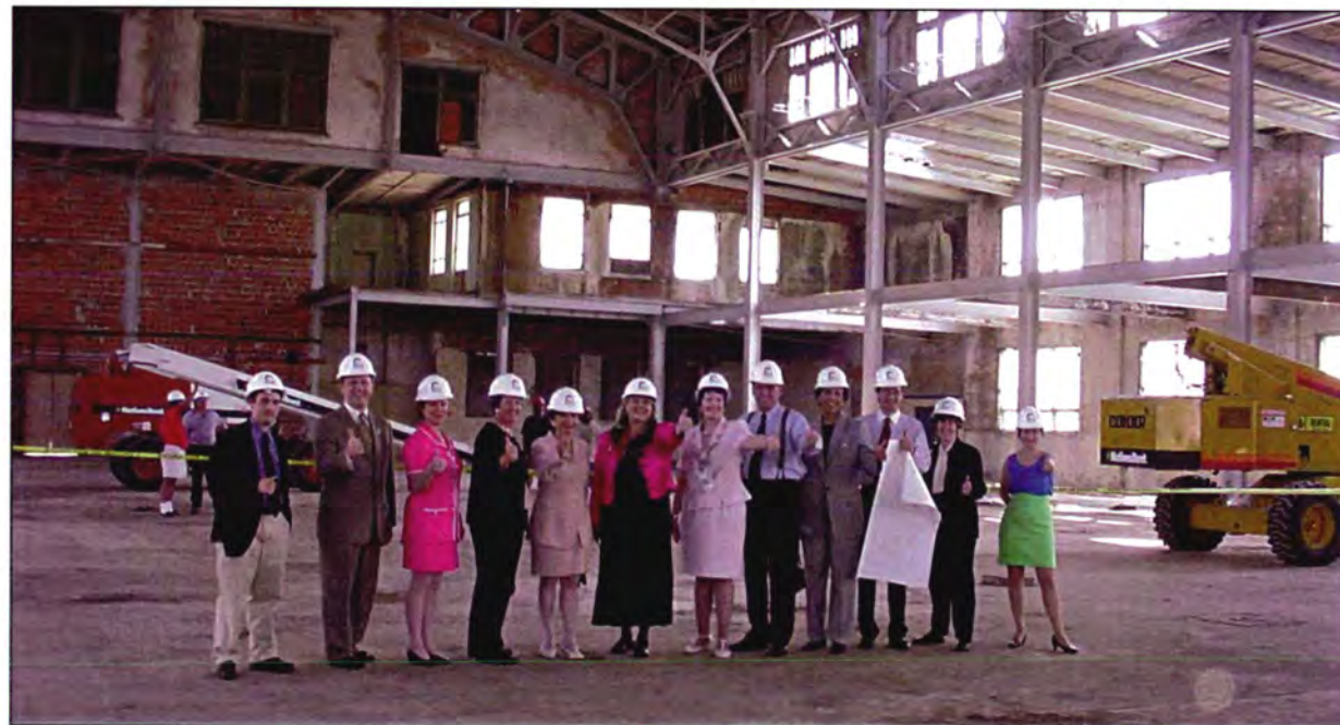
Board members, funders, support- ers and staff members tour the construction site after a board meeting.
