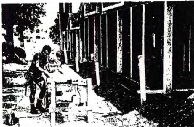
Building a Dream. A craftsman works to ready new townhomes targeted for low-income citizens as part of the Parkside project in Washington. The project is funded by the AFL-CIO's Housing Investment Trust and includes Housing Development Action Grant money from HUD.
