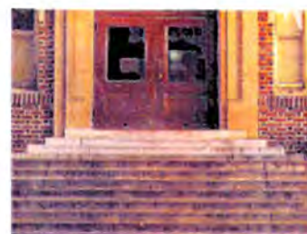
Stairs are a barrier for some.
