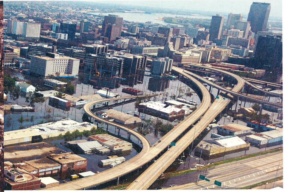
I-10 at US90 Interchange, New Orleans, LA
