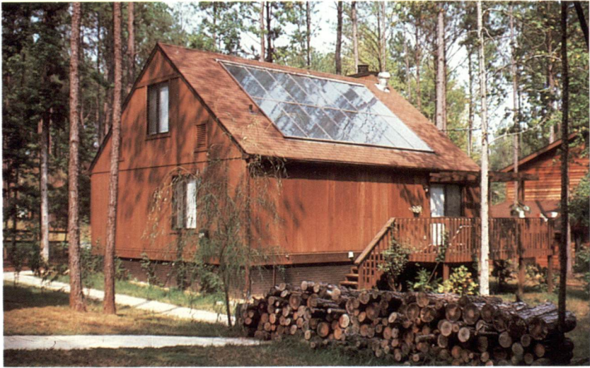
Solar power provides hot water and heat for this home in Shenandoah, Georgia.
